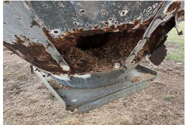
A fiber glass silo doesn't corrode! Salt and ammonium in the feed, combined with water condensation, results in chemical corrosion, to which composite materials are resistant.
